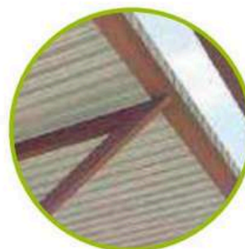
Metal structure from the roof
